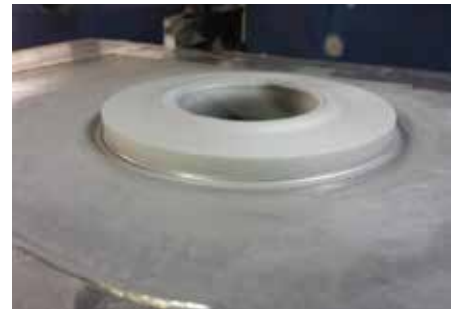
Figure 10. Repaired external corrosion surfaces of the aluminum actuator post.
