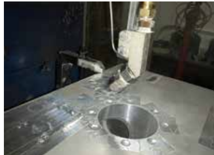
Figure 3. Experimental Setup to repair the valve actuator.
